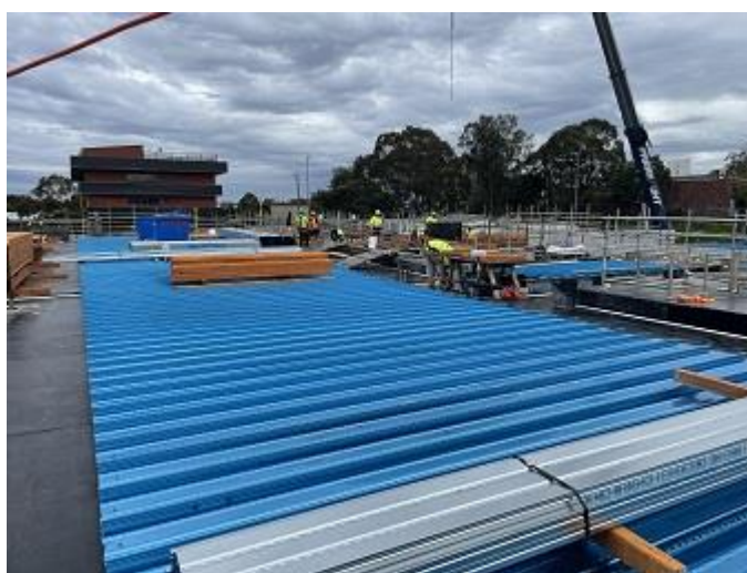
Blackburn Square Shopping Centre Stage 2 (Roof Development Progress), North Blackburn, VIC
