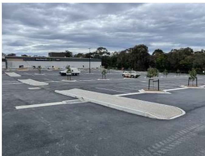
Blackburn Square Shopping Centre Stage 2 (Carpark Development Progress), North Blackburn, VIC
