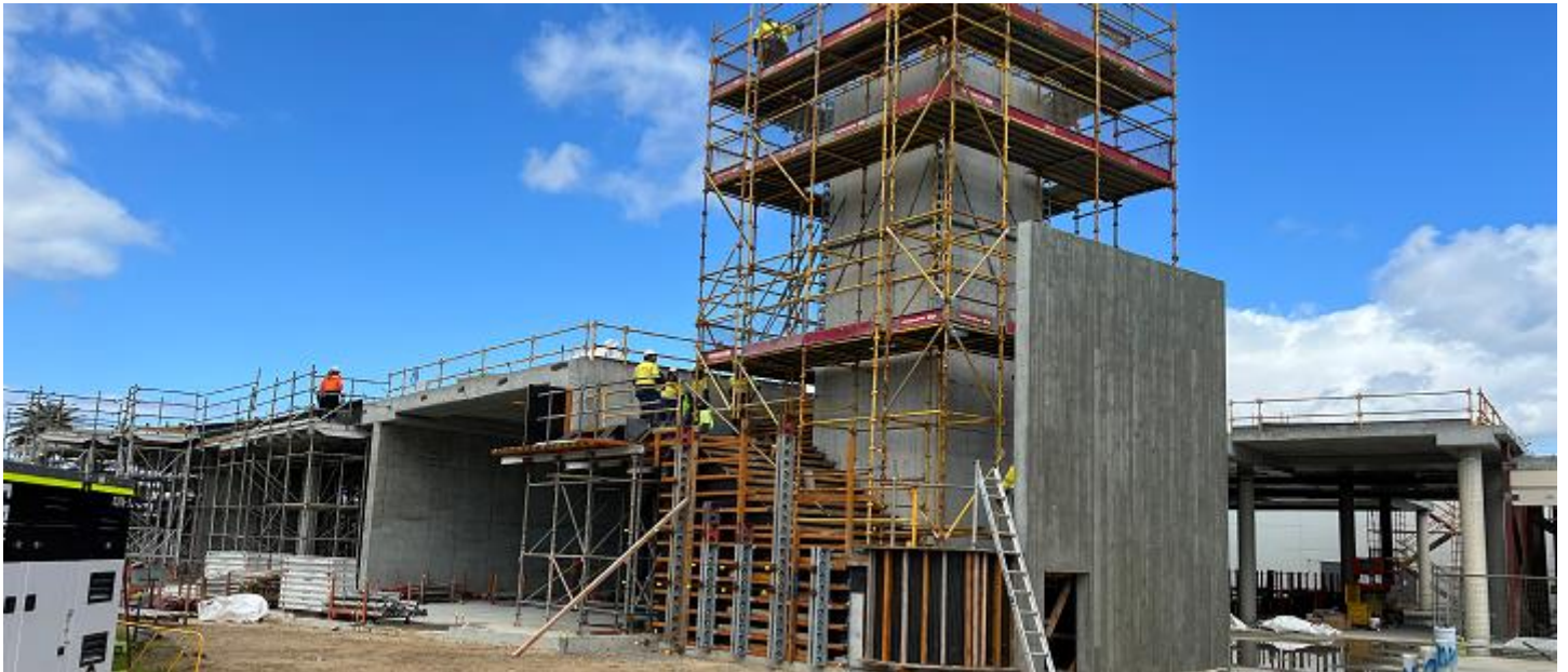
Busselton Central Shopping Centre Stage 3, Busselton, WA
