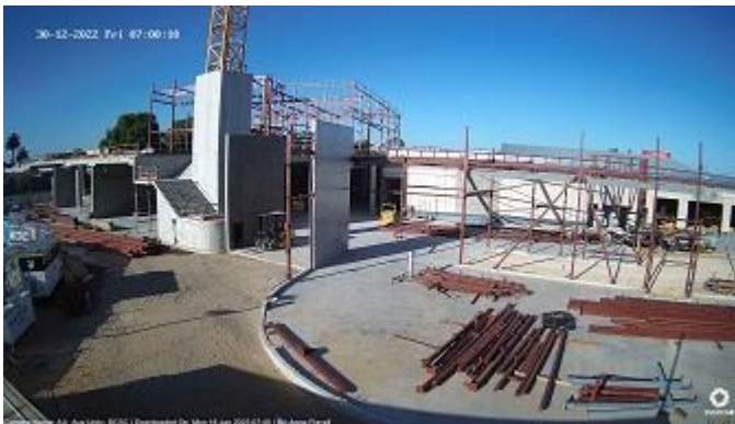
Busselton Central Shopping Centre Stage 3, Busselton WA
