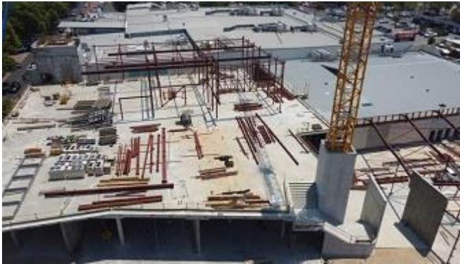
Busselton Central Shopping Centre Stage 3, Busselton WA
