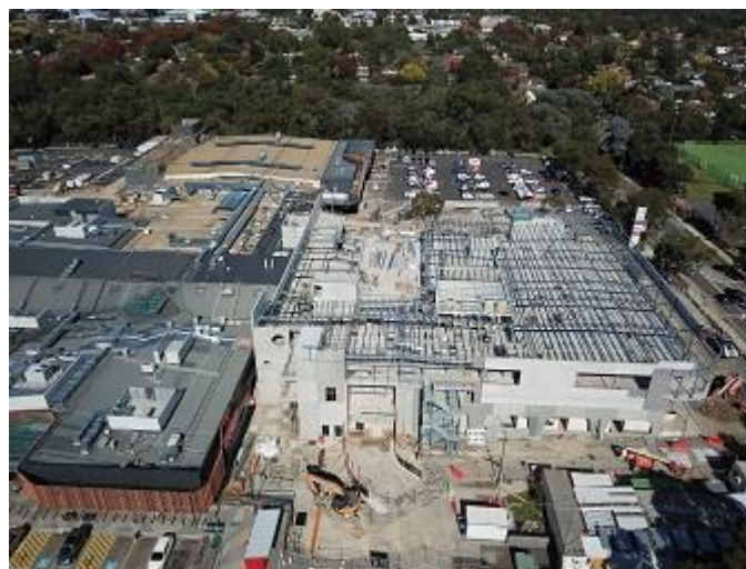
Blackburn Square Shopping Centre Stage 2, North Blackburn, VIC
