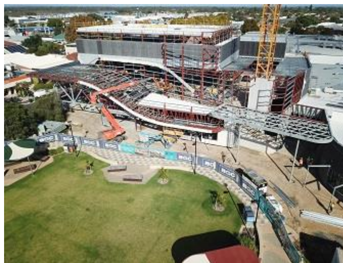
Busselton Central Shopping Centre Stage 3, Busselton WA
