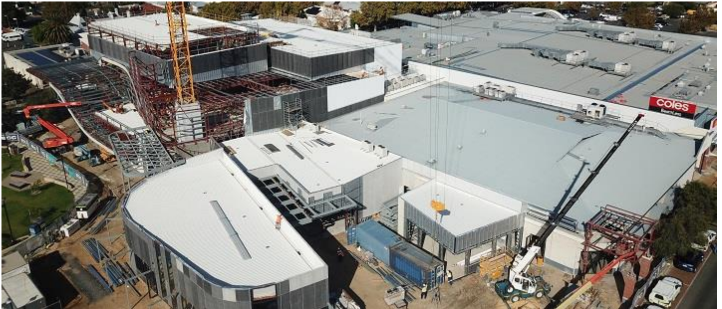
Busselton Central Shopping Centre Stage 3, Busselton WA
