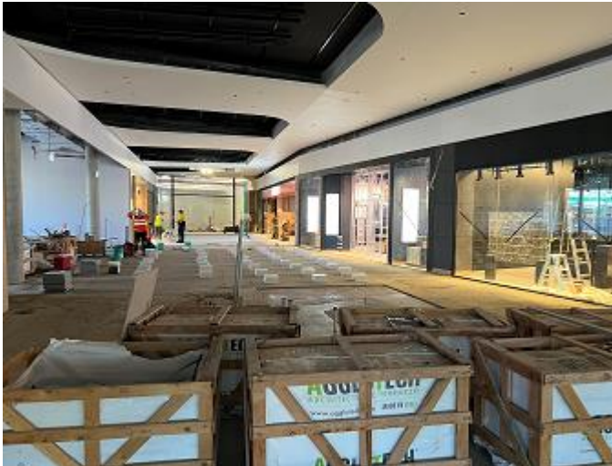
Busselton Central Shopping Centre Interior, Busselton WA
