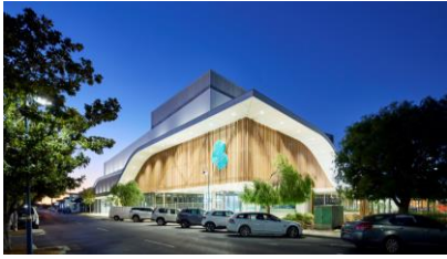
Busselton Central Shopping Centre, WA Coles, Redeveloped 2023
