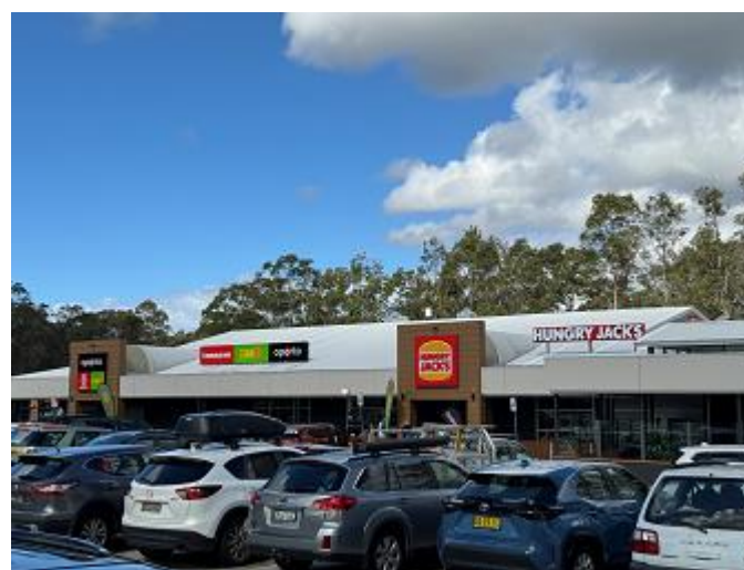
Wyong Twin Service Centres
