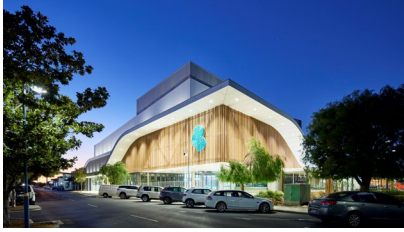
Busselton Central Shopping Centre, WA Coles, Redeveloped 2023
